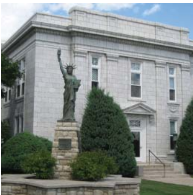
City Hall is a key destination anchor within the Downtown Core.
