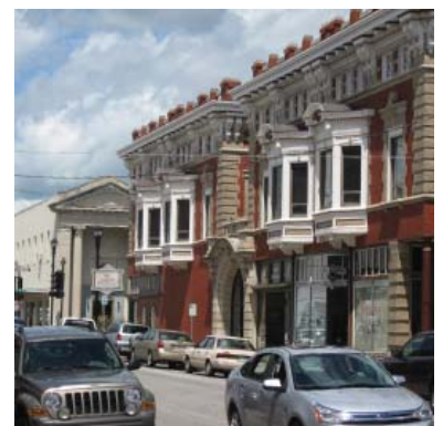
Preservation and enhancement of the historic character of the Downtown Core is a key philosophy of the master plan.
