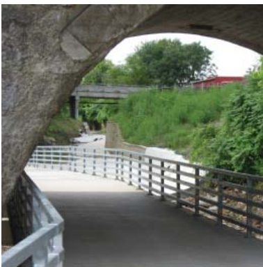
Recently completed in 2009, the 3 Mile Creek and boardwalk provide enhanced connectivity between Haymarket Square and the riverfront.
